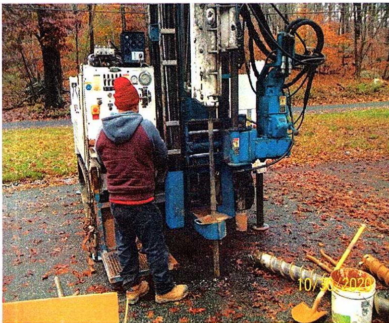
Sample procurement using split spoon samplers and augurs
